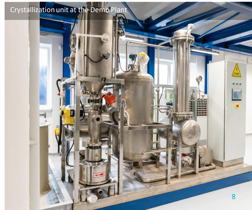
Installation of the Demo Plant
