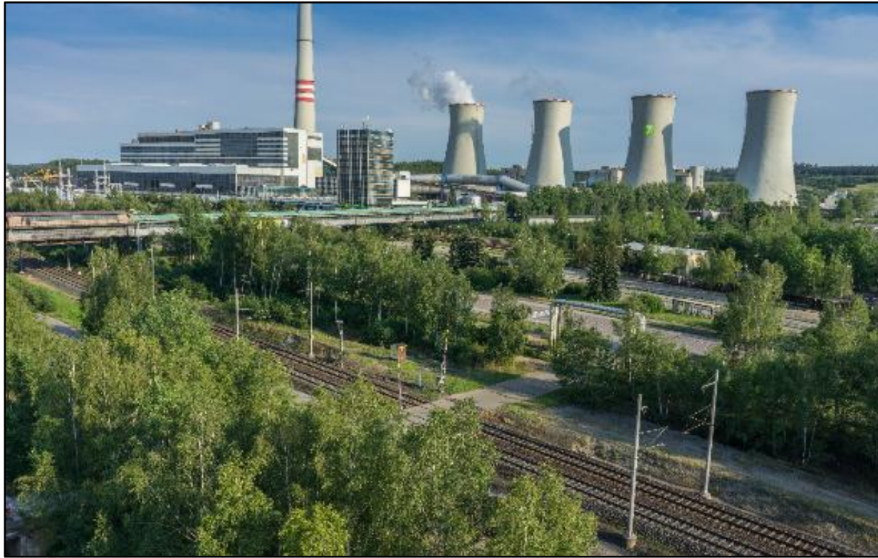
Figure 6-3: Current Power Plant
