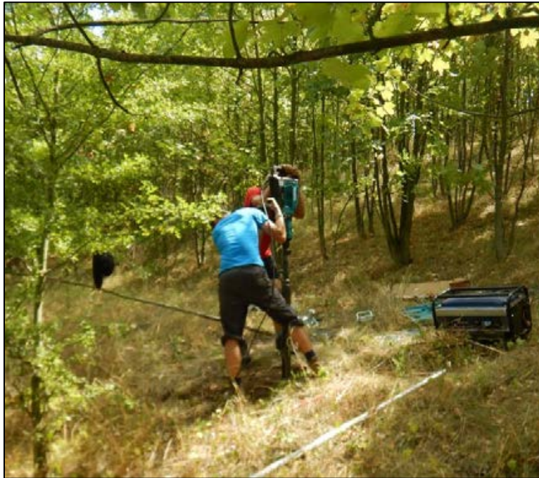
Figure 10-4: Drilling of Perimeter Embankment Hole using Hand Portage Percussion Drill
