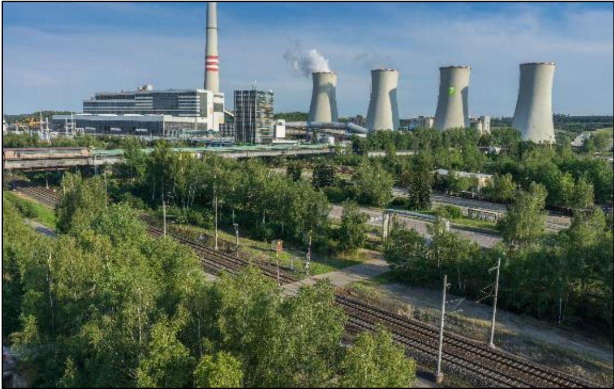
Figure 6-3: Current Power Plant
